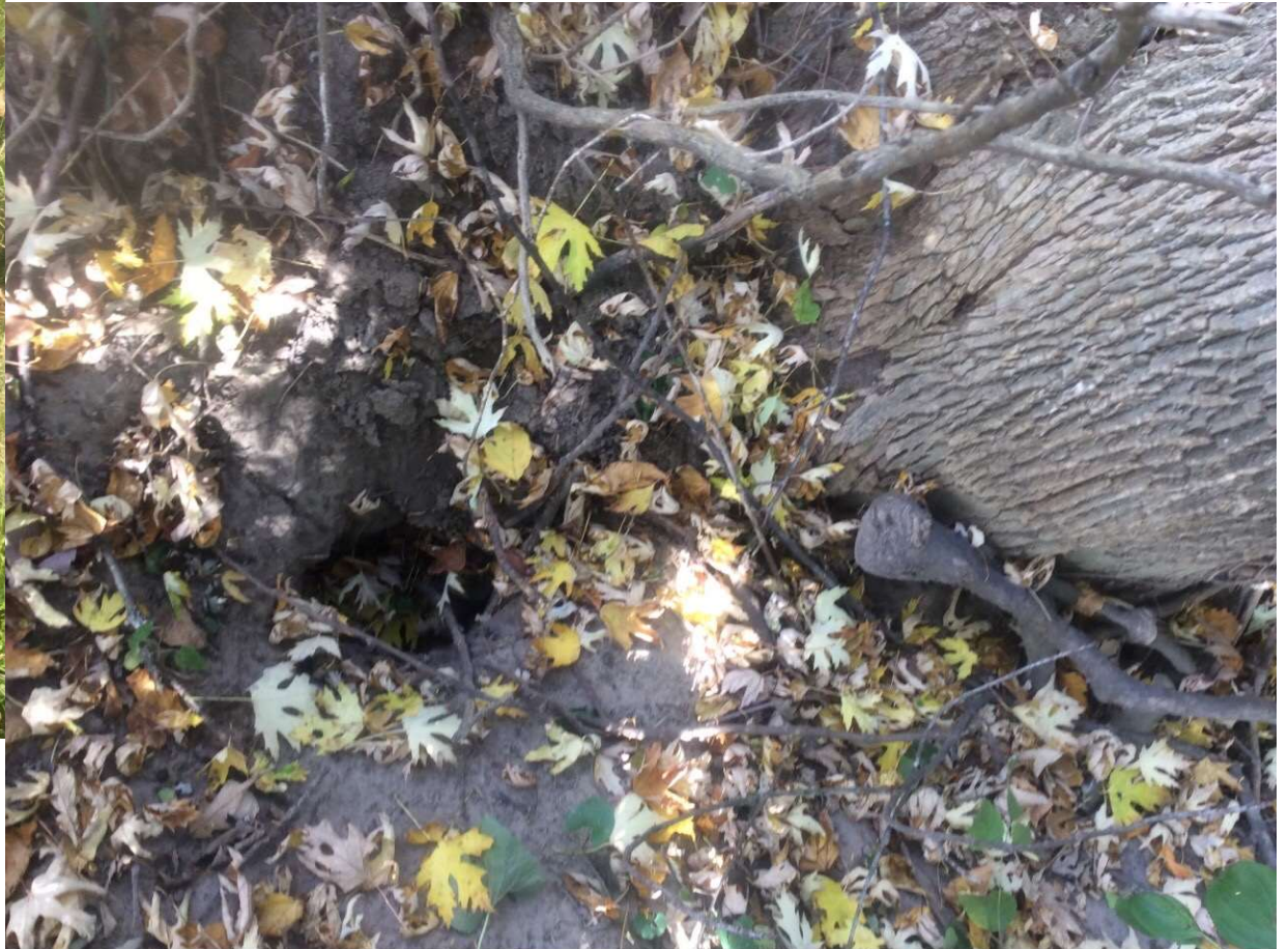
Sink hole along the route of the Gradt Tile Drain
