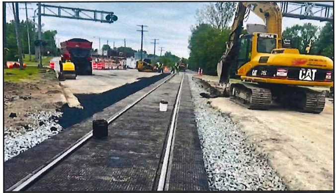
Dixie Hwy (Elmport & Prospect) - Bridgeport Twp Railroad Crossing Reconstruction
