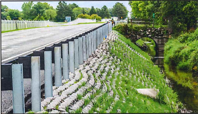
Kochville Rd (West of Davis) - Kochville Twp Guardrail Replacement & Bank Stabilization
